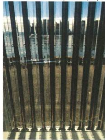
Figure 6. Appearance of solar hot water tubes, which will be present behind the glass wind screens on the south and west sides of the building's crown.
