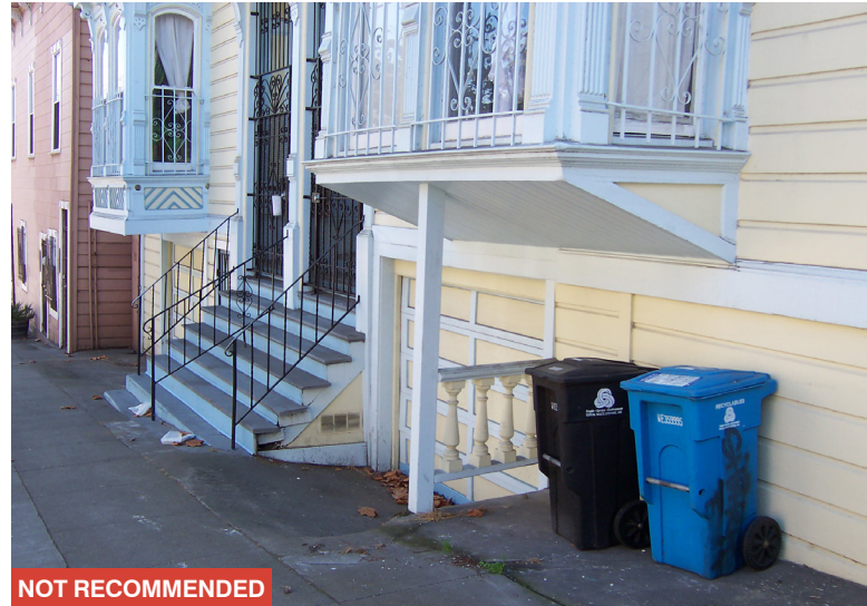
The base of this historic projecting bay was adversely impacted for this garage. This treatment does not meet the criteria for inserting a garage within an existing structure.
