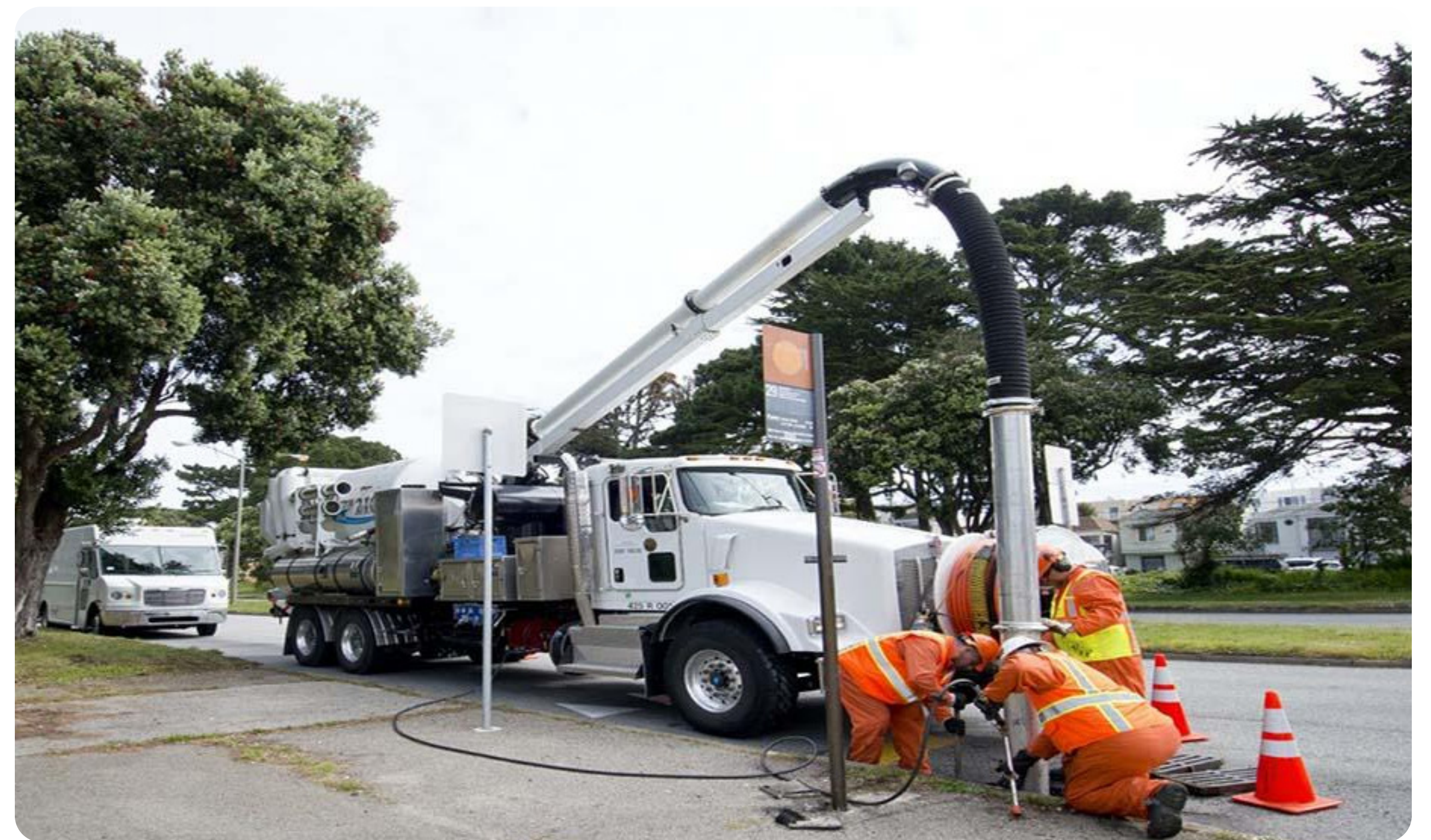
Sewer maintenance - Sunset District. Photo: SF Public Works
